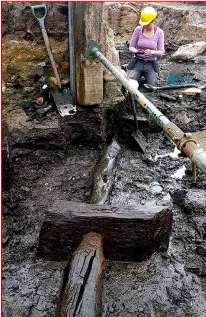
Fig.11. Water pipe found on the borders of England and Scotland.
